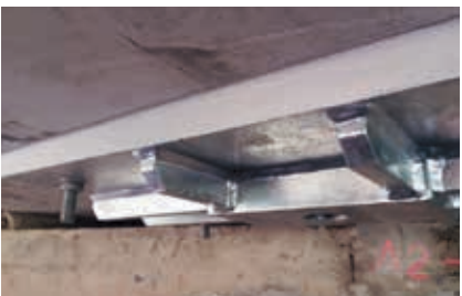
補強部材隙間充填
